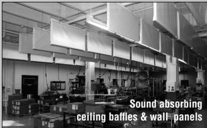
Sound absorbing ceiling baffles & wall panels
