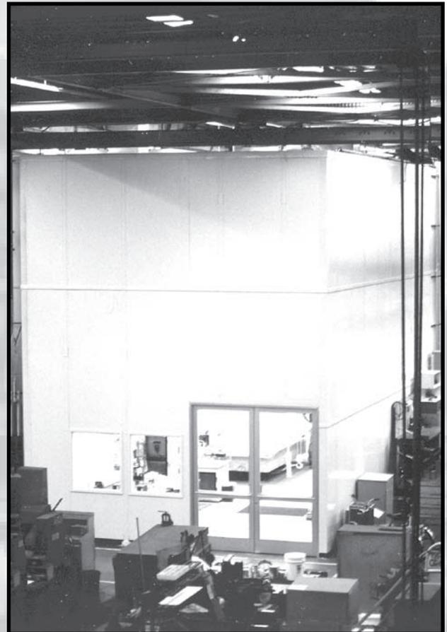
Temperature gradient within 20'-0" cleanroom is maintained at  $\pm 1^\circ$  F over one meter.
