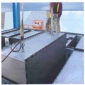
AN INNOVATIVE SILENCER CONCEPT DESIGNED FOR USE IN APPLICATIONS WHICH REQUIRE HIGH VOLUME FLOW RATES. SELF-SUPPORTING DESIGN, IN EITHER HEAVY DUTY ALUMINUM OR STEEL CONSTRUCTION, MINIMIZES STRUCTURAL REQUIREMENTS.
