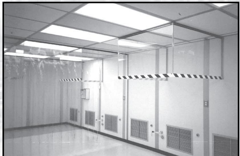
Multiple cleanroom classifications are established within the same building envelope utilizing clear vinyl softwall panels.
